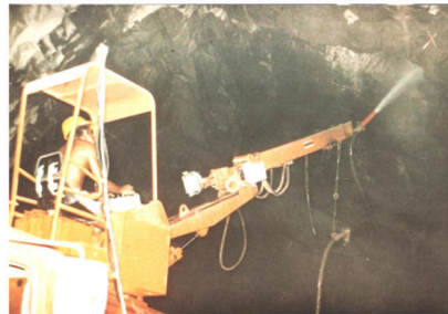
Figure 9 Shotcrete spraying process using 'roboshot' (Hoek, 1993)
