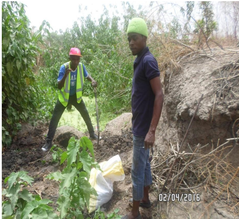
Plate 1: Location1: Malero, Depth of 3.2m Medium to Coarse Sand.
